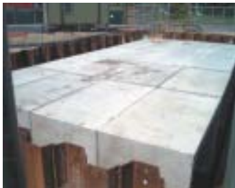
▲ Hanson box culverts in use at Heathrow Terminal 5 project.
