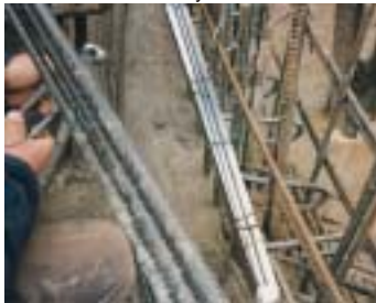
▲ Use of Stabox® in curved sliding formwork.
