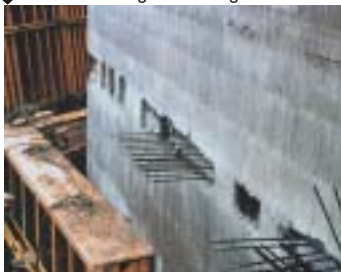
◆ Non obstructing to climbing formwork.
