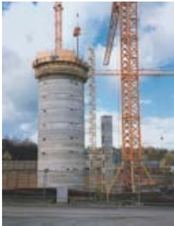
▲ Walls and floors tied to circular structure.
